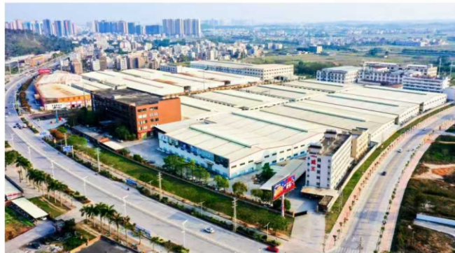
Guangdong Weking Group Co., Ltd (Headquarter located in Zhanjiang, Guangdong)
